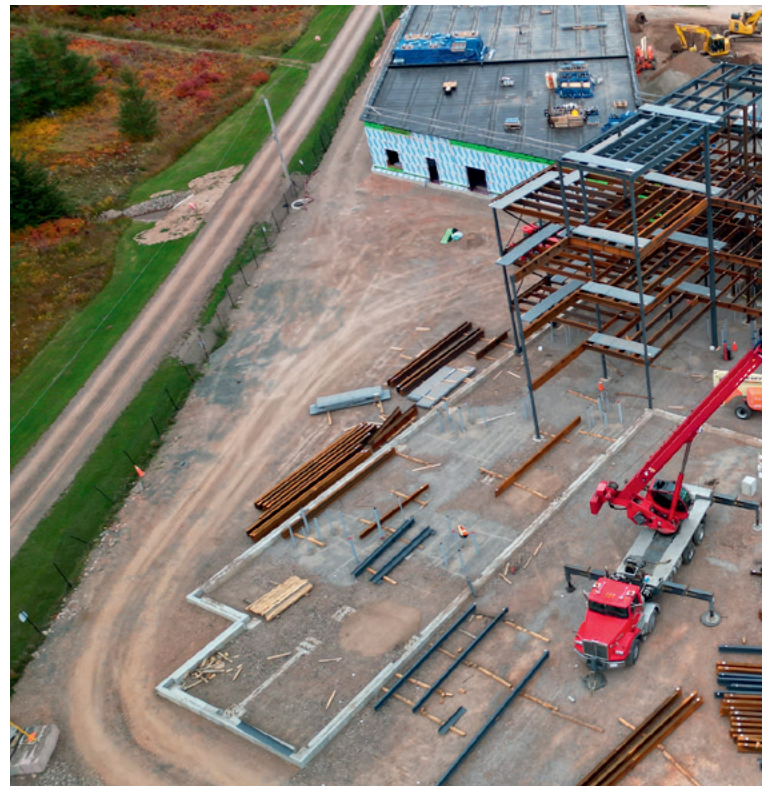
Construction site throughout October 2025. (Photos: Lindsay Construction Ltd.)
