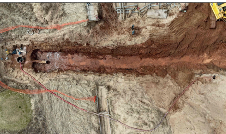
April 22 (morning): Final trench excavations were completed, and the old section of the outfall pipe was removed.
