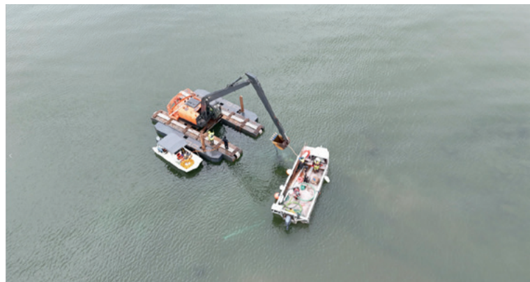
April 14: The amphibious excavator holds the end of the outfall pipe in place while divers check the depth and position of the pipe.
