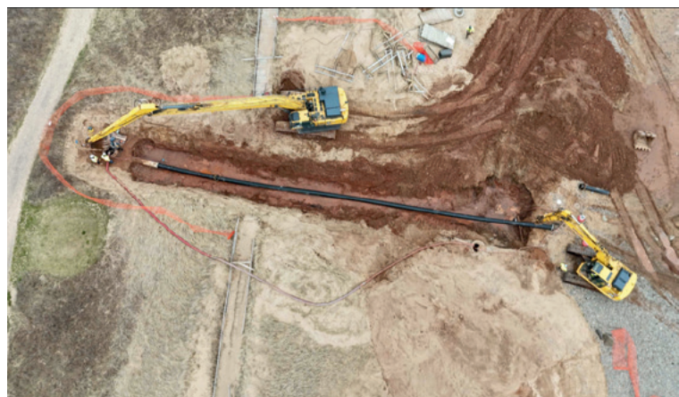
April 22 (afternoon): The new section of pipe was lowered into the trench. The inland side (left) was connected to the manhole, while the seaward side (right) was tied into the newly installed marine portion of the outfall system.
